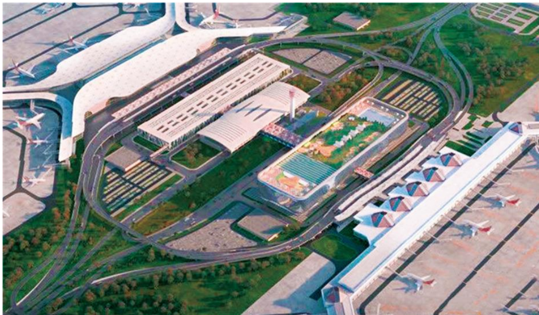
Figure 1. Comprehensive transportation center of Haikou Meilan Airport
