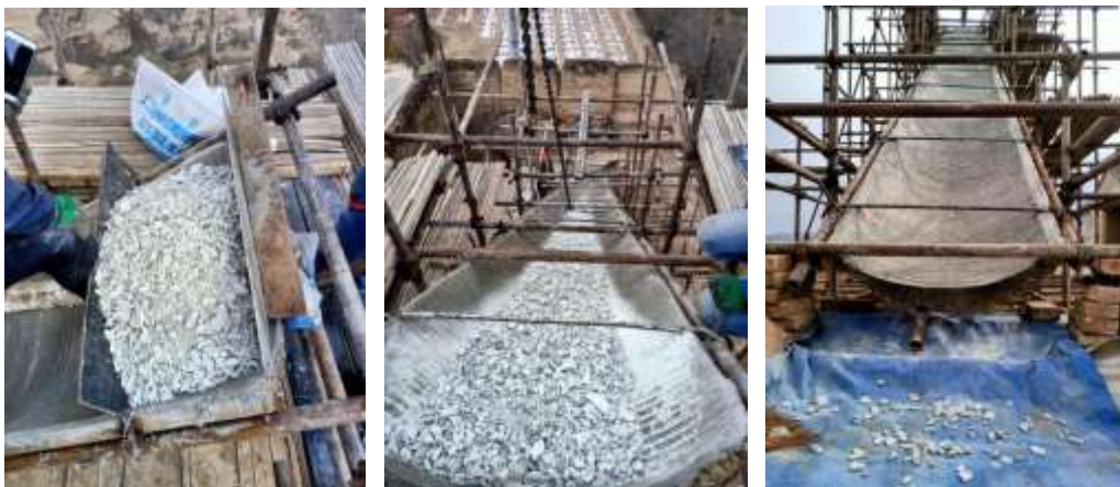
Fig 4: Slag discharge process diagram
