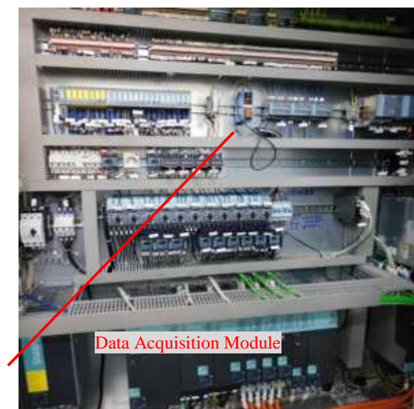
Fig 1: Internal wiring of gear hobbing machine
